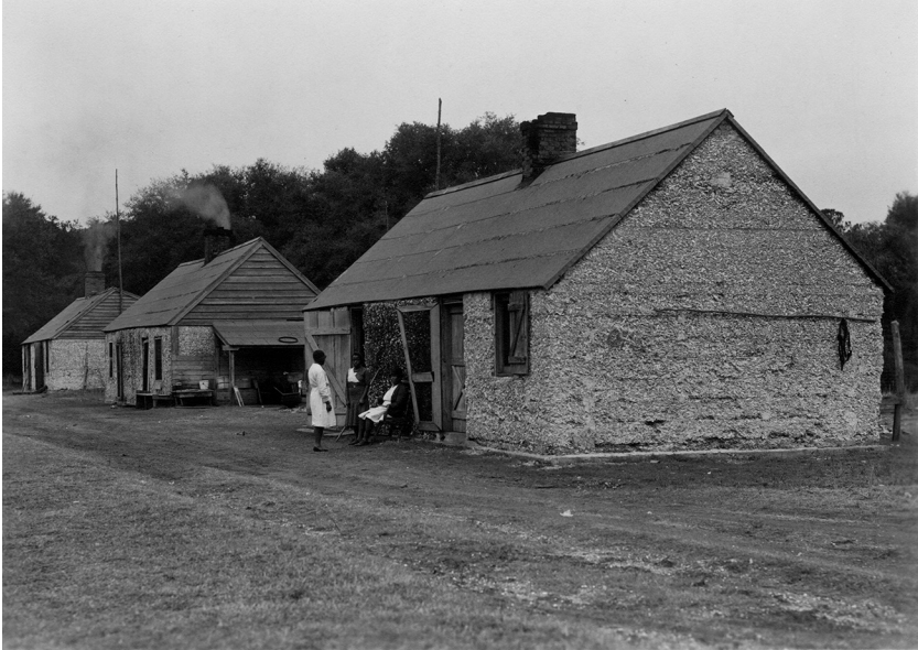
Tabby cabins on Ossabaw Island, circa 1930s. Originally built for enslaved people in the 1840s, the cabins probably stood where huts were erected during the 1760s for the first captives. Courtesy of Georgia Historical Society.
